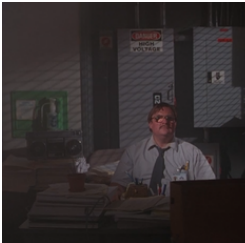
An ex-employee of Initech sits in the basement of the building. One of the signs behind him reads “Danger high voltage”. This is not a physically comfortable environment.
